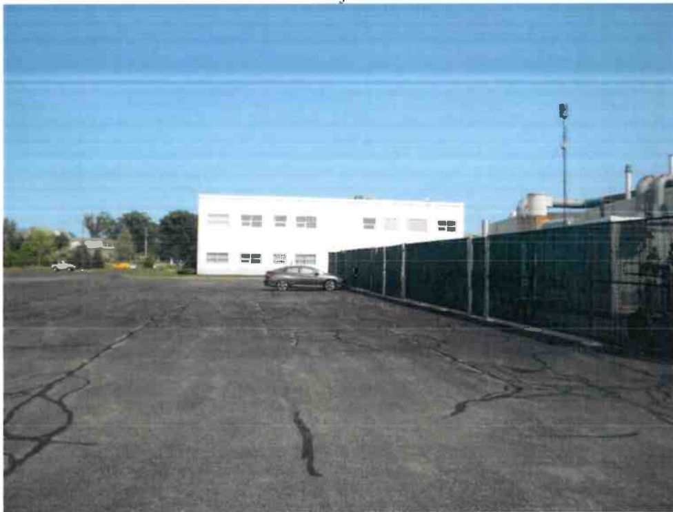
Rear of Subject Section & Office Section
