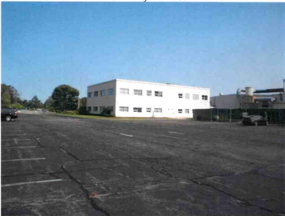
Rear of Office Section
