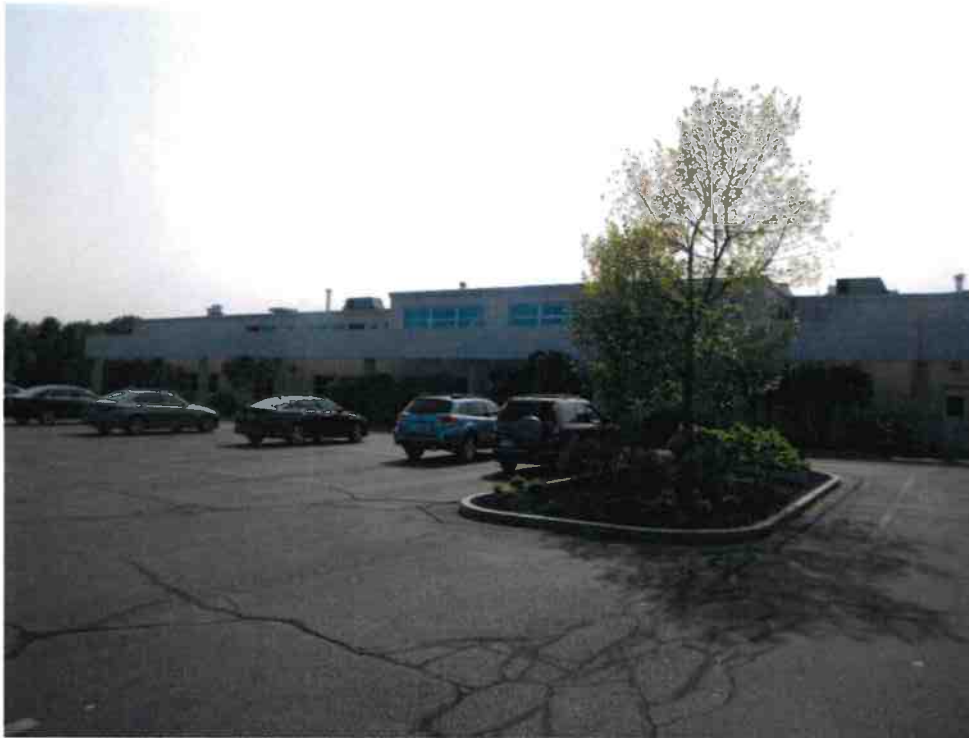
Front of Subject Section
